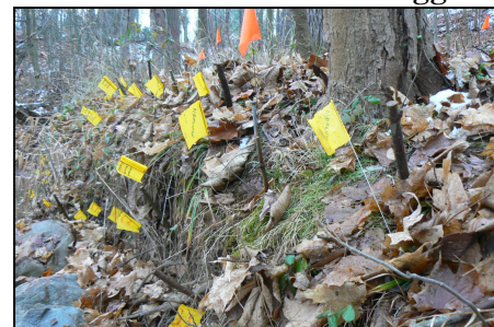
Live stakes installed and flagged
