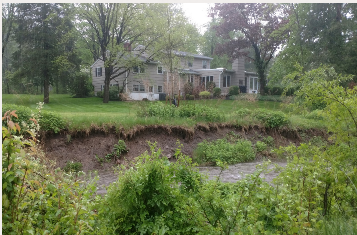
Erosion forms along an unbuffered stream bank.
